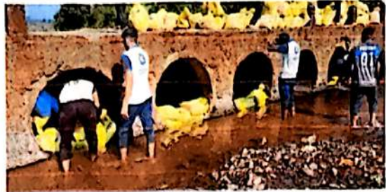
Constructed Vanrai Bandhara on Arjuna river
